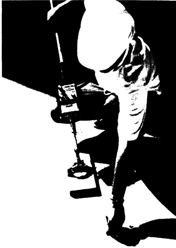
Figure 29. Prior to placement of any anode system, the deck should be checked for thin cover areas.
