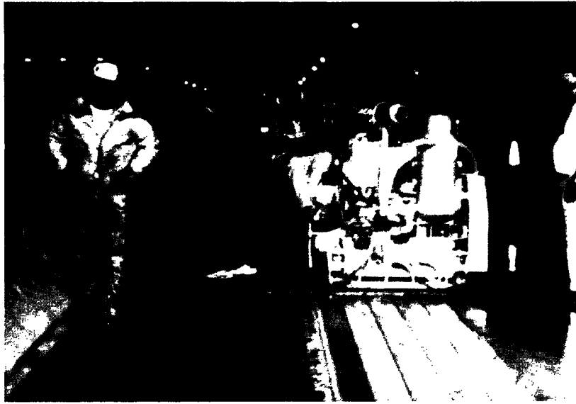
Figure 33. This heavy-duty machine can cut up to five slots in one pass.
