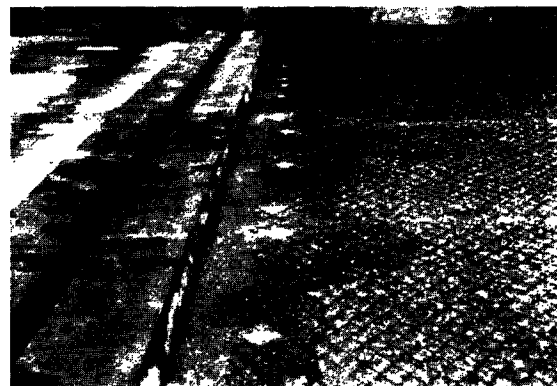
Figure 59. The mesh panels are stopped approximately 3 in. from the metal expansion joint.
