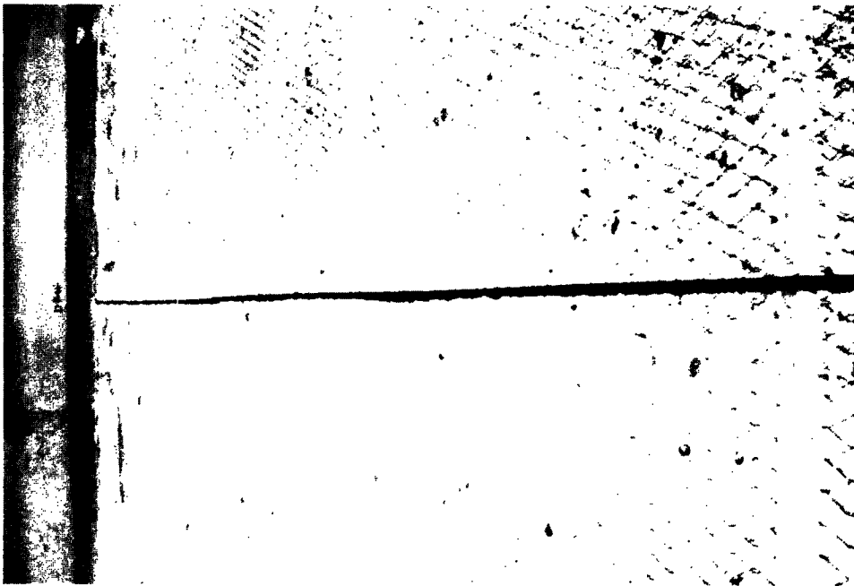
Figure 60. The transverse conductor bar electrically connects the 4-ft.-wide panels together.
